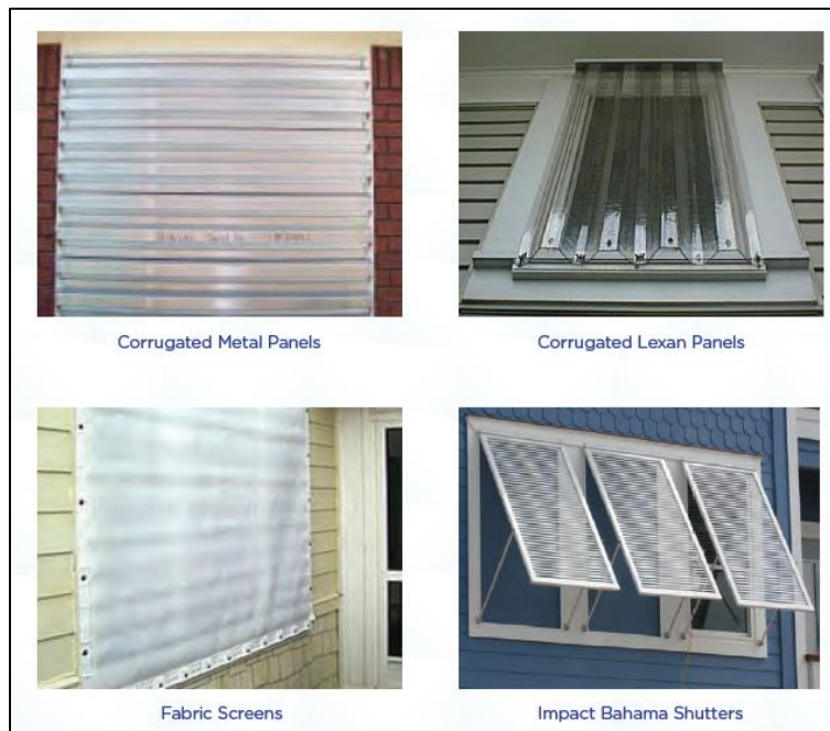
Examples of Shuttering Systems
